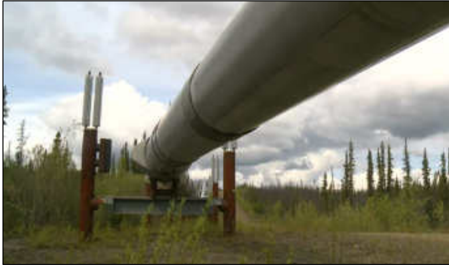
Abbildung 30: Alaska Pipeline mit Heatpipes ( As permafrost thaws, protecting infrastructure becomes more important, 2021 )
